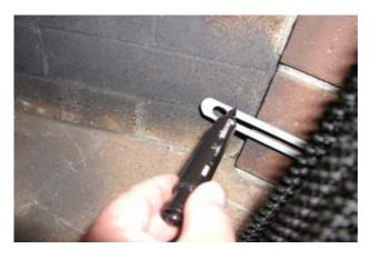
**STEP 6** Using a 5/16" masonry bit, drill hole where marked.
